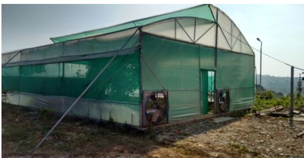
Fig. 1: High-tech green house
